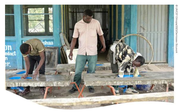
Gezahegn Melese, the team leader for communicable disease prevention and control, providing technical support, so the toilet made with cement slabs are built properly. "The toilets were unimproved and made of mud, but now we build it with cement so its easy to clean and sustain," says Gezahegn Melese.
