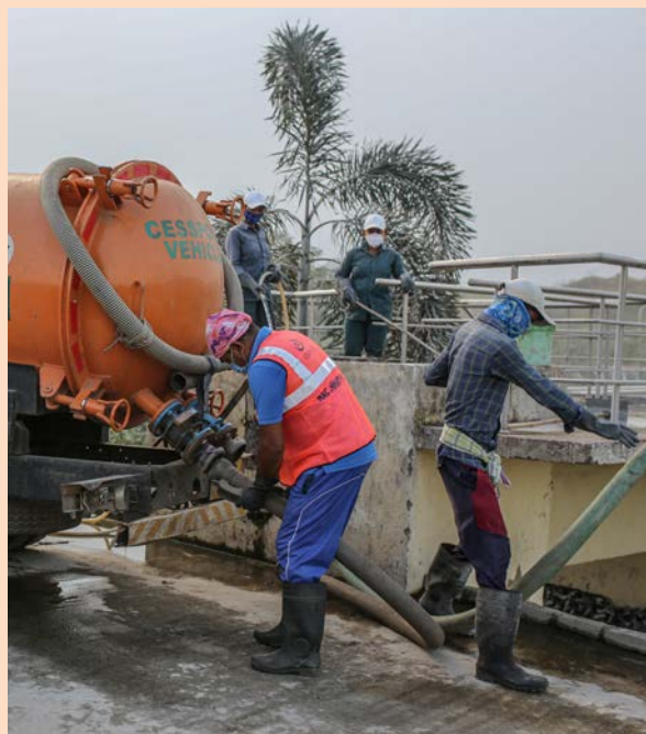
Swachhta Saathi unloads faecal sludge using a Cesspool vehicle inside a Faecal Sludge Treatment Plant (FSTP) at Ganjam District in Odisha.
