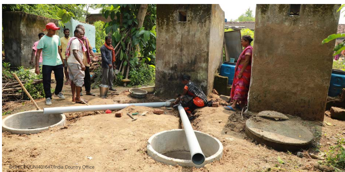
Toilets are being retrofitted in Odisha.
