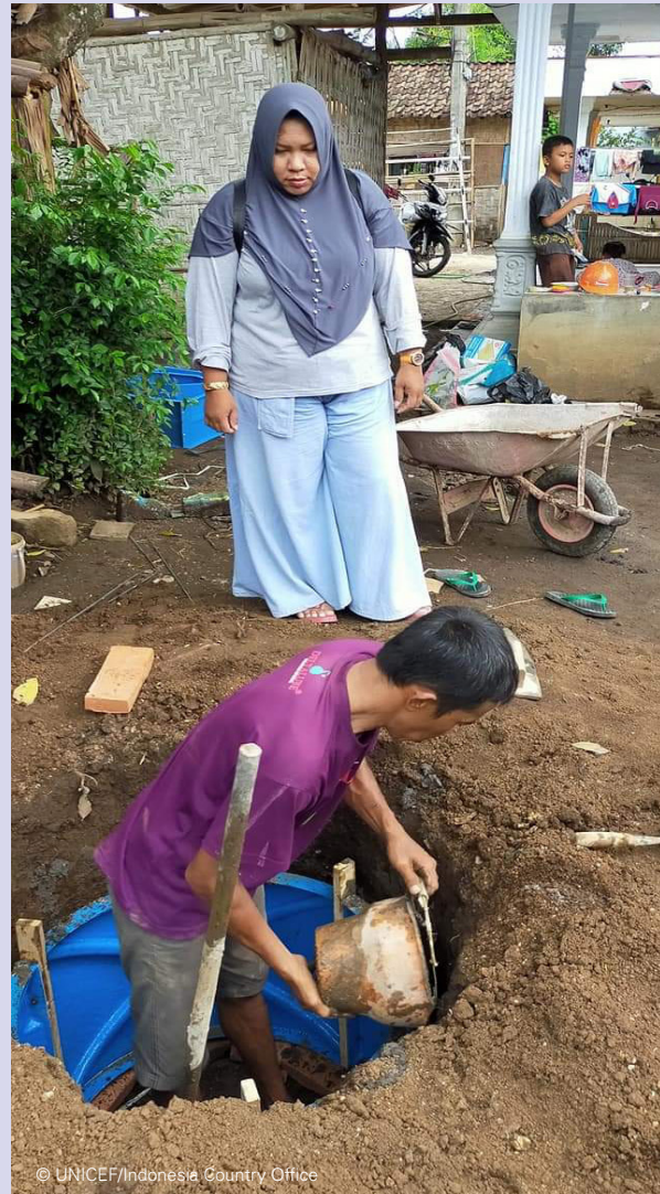
Dewi observes the construction of a septic tank in Lumajang.
